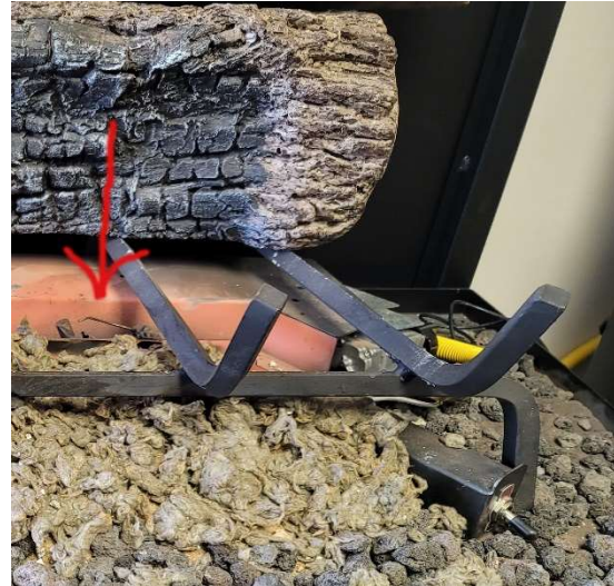
Figure 2 – Arrow pointed at pilot assembly with logs removed
